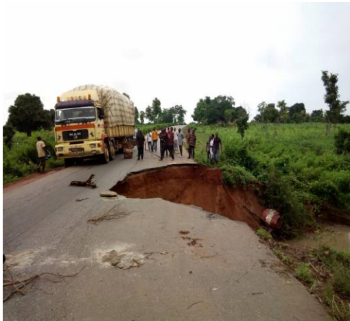
Picture 9. Jos – Abuja Road
